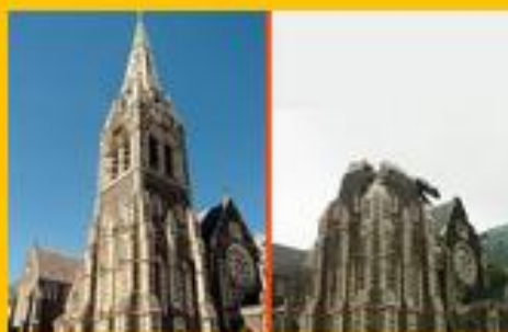
The left, my photo, but it's taken in my hometown. It's of the Christchurch cathedral, before and after the February 22nd earthquake in 2011.
